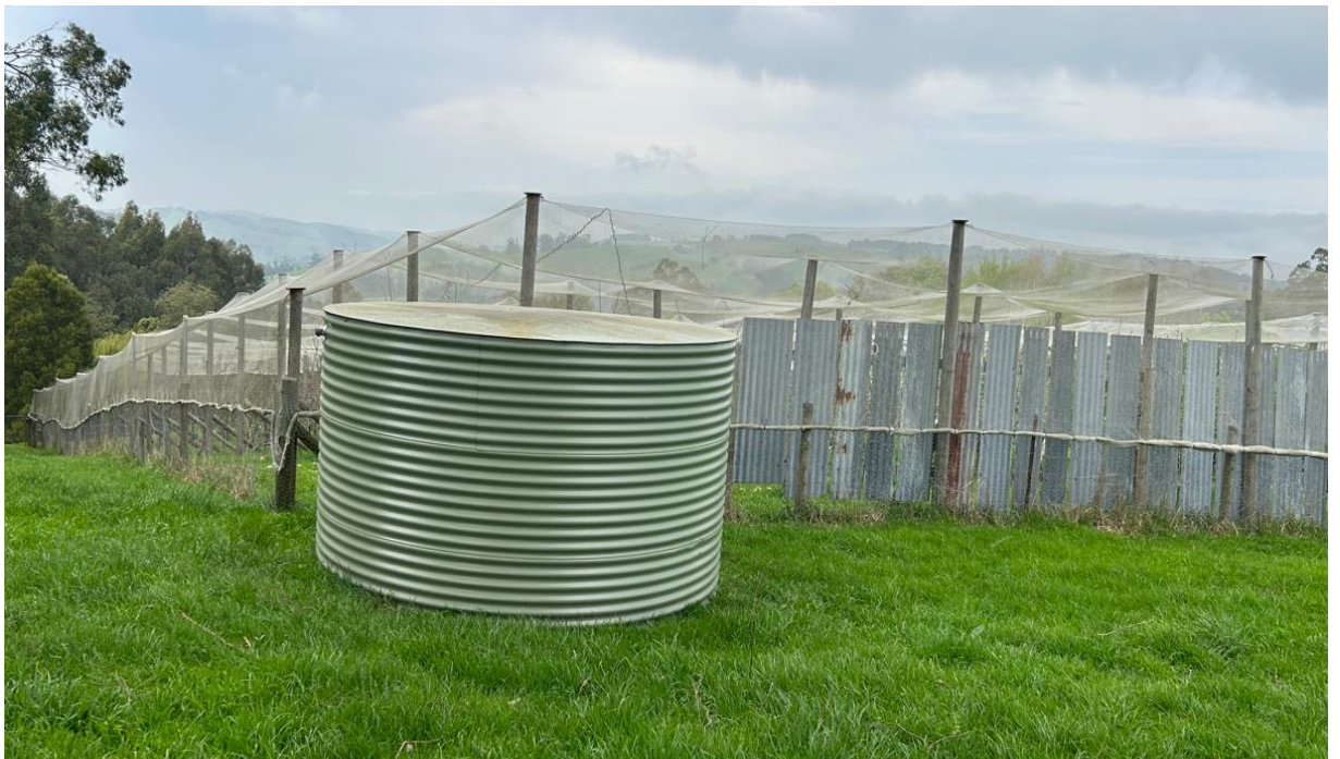
Image 13 –water tank fed from the dam.
