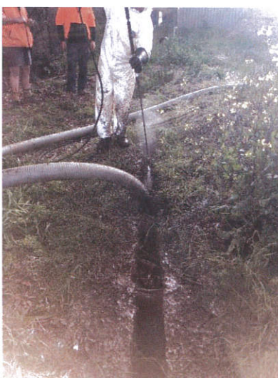
Hydro-excitation uncovered significant roots (60mm dia.) up to 4.5m from the base of the tree
