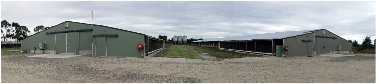
Figure 4. Evaporative Cooler Pads – Sheds #9 and 10
