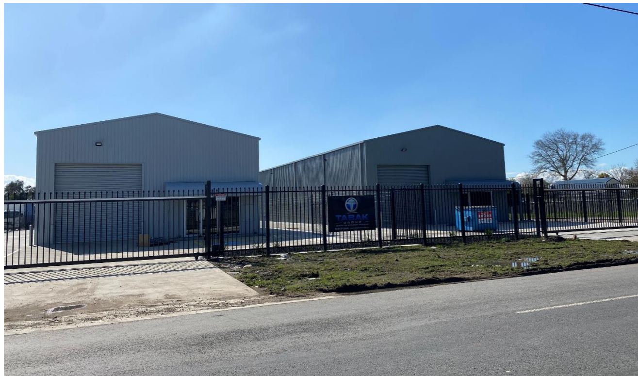
New industrial developments on Waterloo Road have substantial setbacks with landscaping and carparking incorporated.
