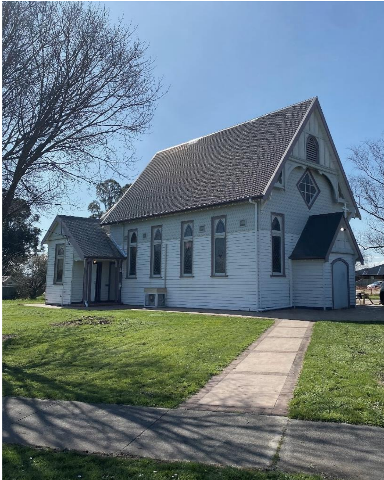
St Jarlath Catholic Church, Campbell Street (HO14)
