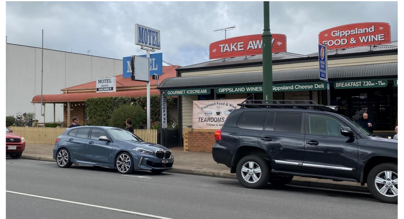
Examples of advertising signage located on or near the front property boundary. The mix of sign types in this example include roof-mounted, pole, banner, and internally illuminated.
