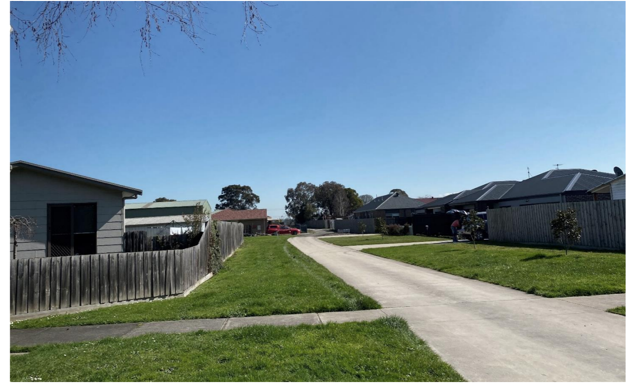
Constructed section of Hanns Lane, located to the east of Loch Street.
