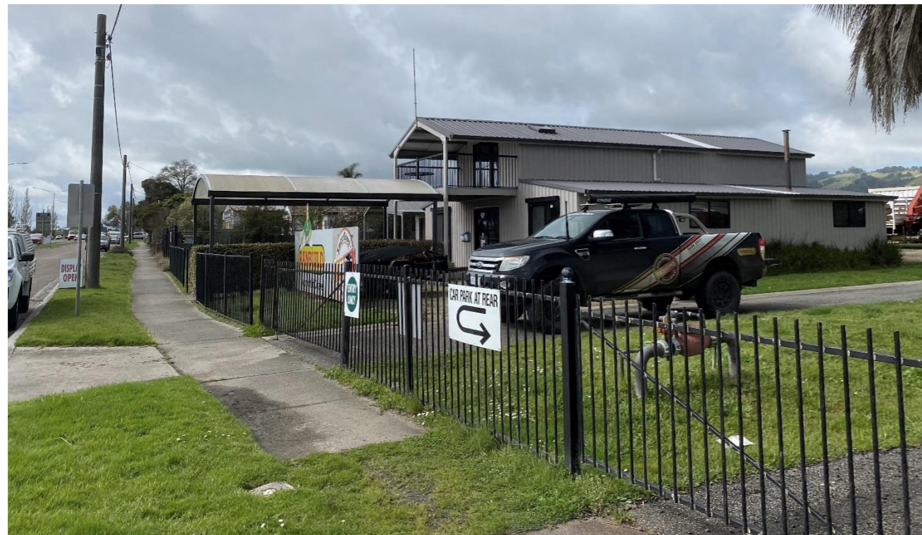
Commercial building construction is typically steel frames with colorbond cladding, which gives this area an industrial feel.
